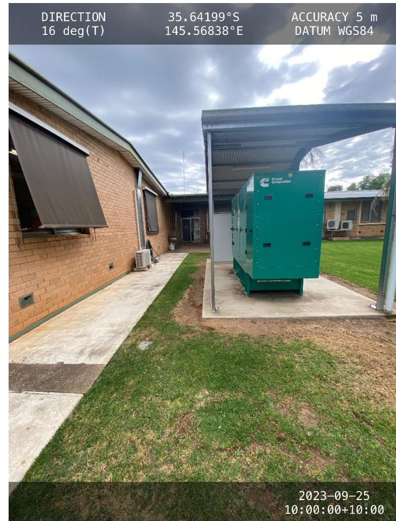
Photograph 4: Current back-up generator
